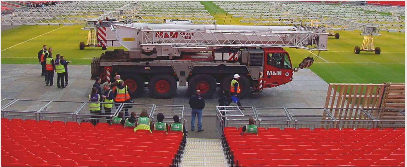
Terratrak system, Wembley Stadium, London
