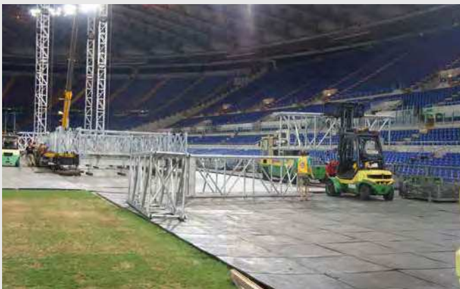
Terratrak product application, Olympic Stadium, Rome
